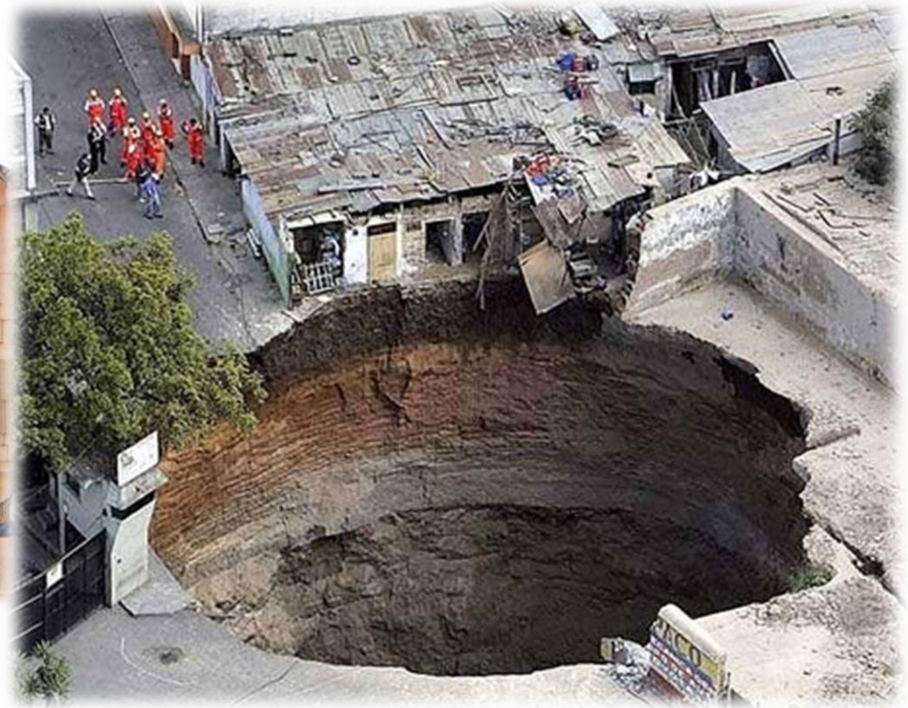
Guatemala City 2007 - 330 foot deep – 7 people reported missing
