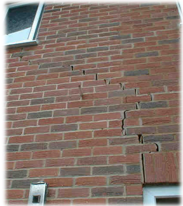
Opposite to Subsidence with tapered stepped diagonal cracking wider at the bottom
