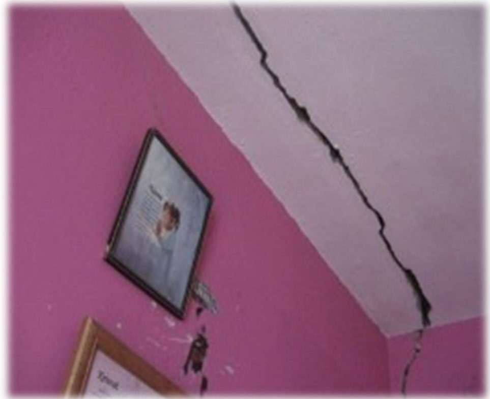
Internal cracking adjacent to bowing wall
