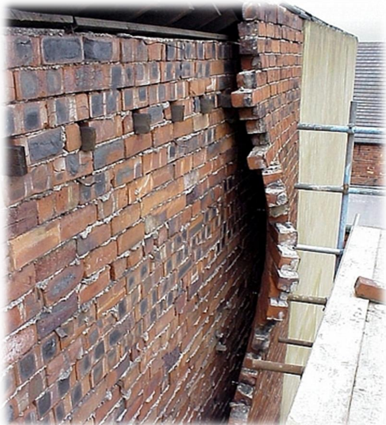
No Wall ties causing bowing and 'peeling'
