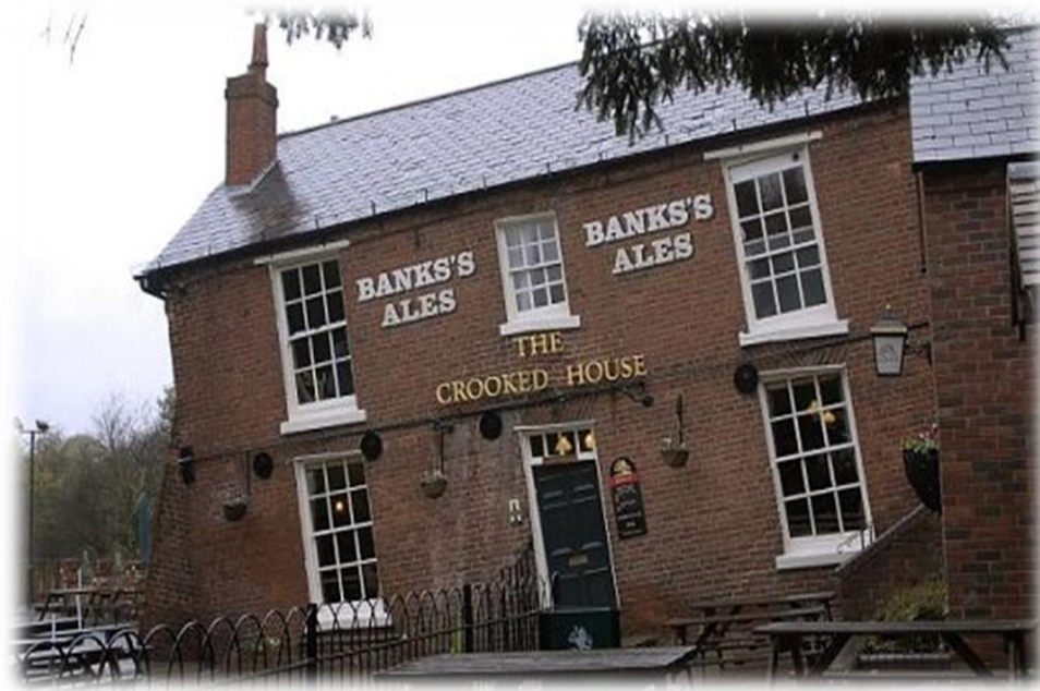
Current view; note lateral restraint and buttresses
