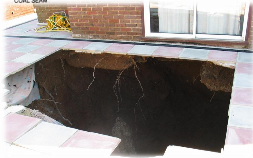
Chalk mine in Hemel Hempstead following the Bunsfield explosion
