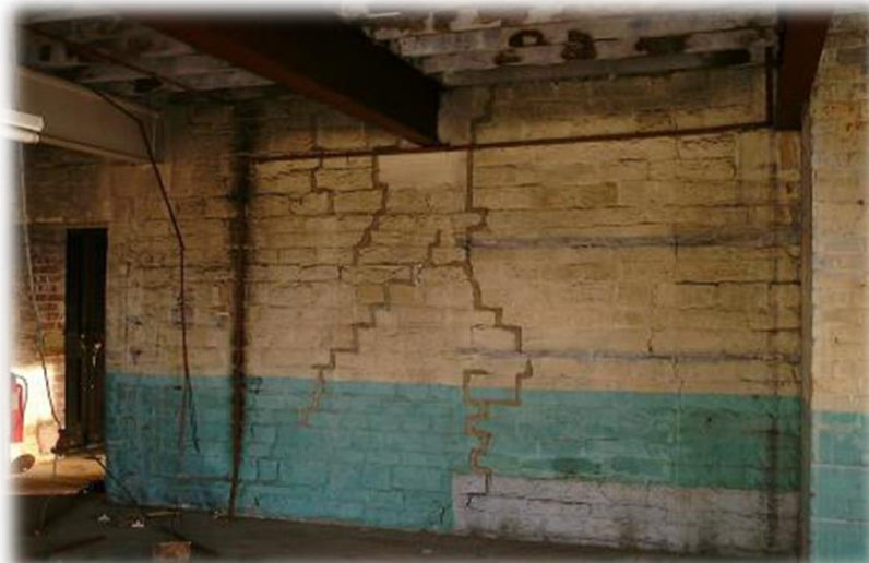
Localised distress to masonry wall caused by built-in floor beam
